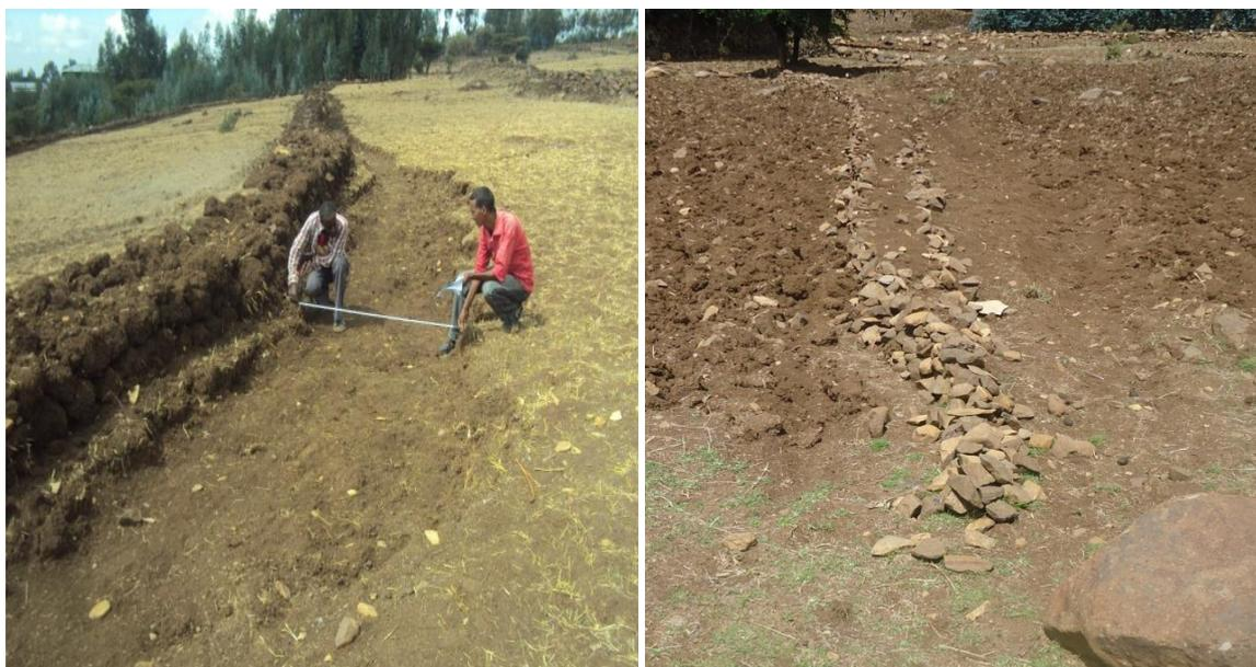
Figure 4: Improper bund channel design
